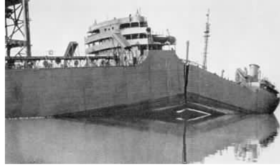
(b) A liberty ship failure
