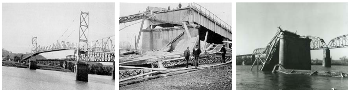
(a) Point Pleasant bridge (b) Point Pleasant bridge after the collapse (c) Point Pleasant bridge after the collapse
